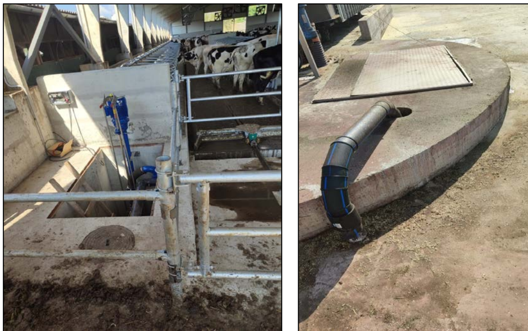
Figure 4 Onsite Manure Collection and Transporting to the Pit
